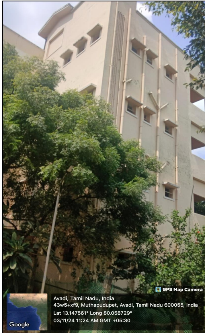
Figure: Water Distribution through Tanks in EEE building.
