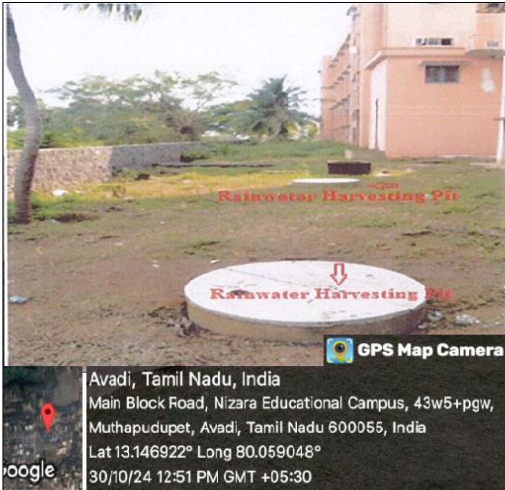
Figure: Rain water harvesting pits near CSE& IT Building
